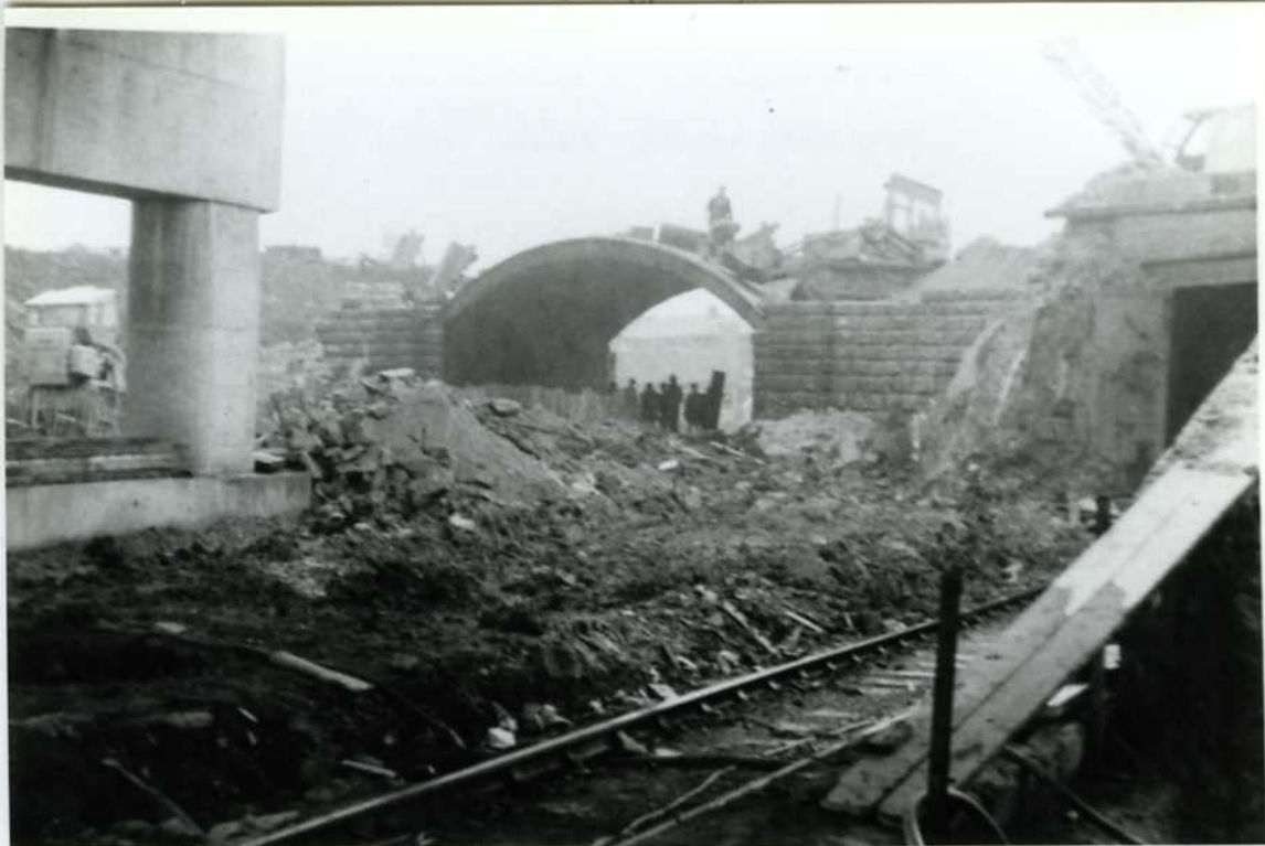
DEMOLITION OF POOL BRIDGE C1959-60 TO REPLACE IT WITH CONCRETE FLY-OVER FOR A184 OVER LEAM LAKE.
