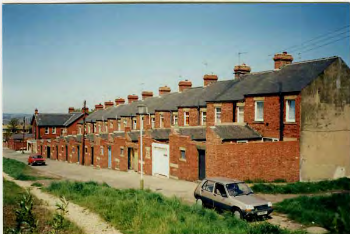
BACK OF EAST VIEW TCE. AT THE BOTTOM CAN BE SEEN THE DETACHED COLLIERY MANAGER'S HOUSE FACING NORTH. ALL THE BACK YARD WALLS STILL HAVE COAL HATCHES AND BELOW THEM ASH CLOSET OPENINGS TO EMPTY SAME.
