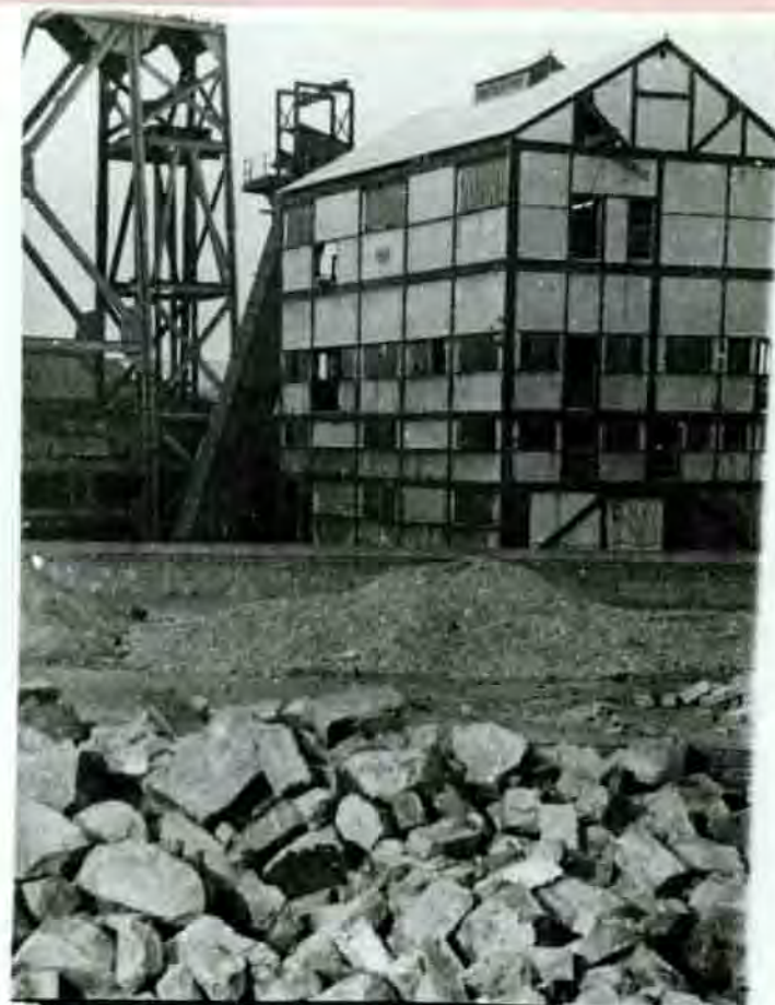
HEWORTH TOWN PIT LOOKING EAST
