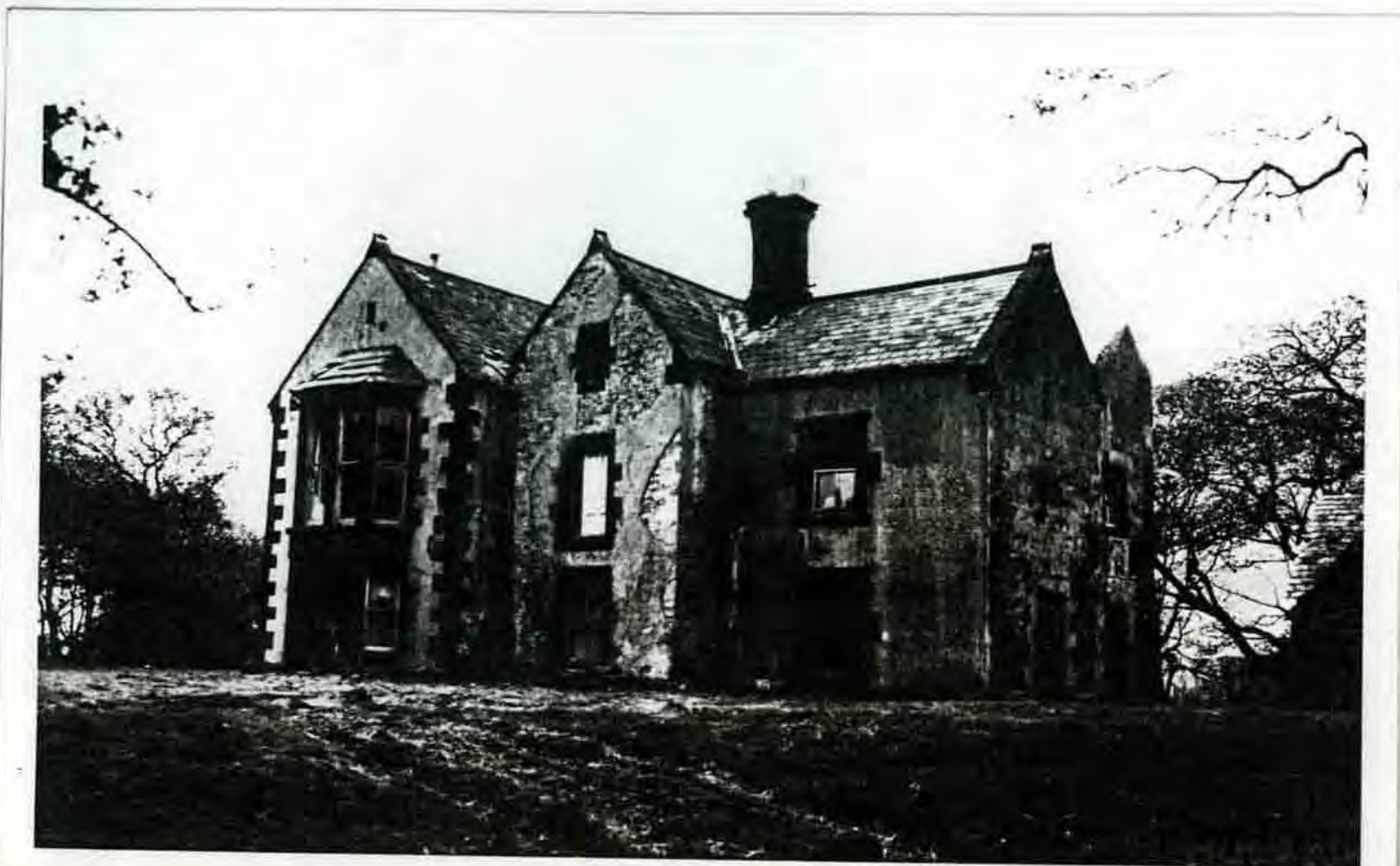
WHITE HOUSE (OLD HALL) UPPER HEWORTH. 17TH CENTURY. HERE DERELICT.
