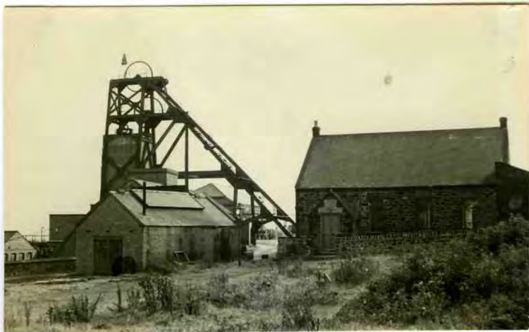
PIT HEAD AND PRIMITIVE METHODIST CHAPEL. DERELICT AND AWAITING DEMOLITION, C. 1963.
