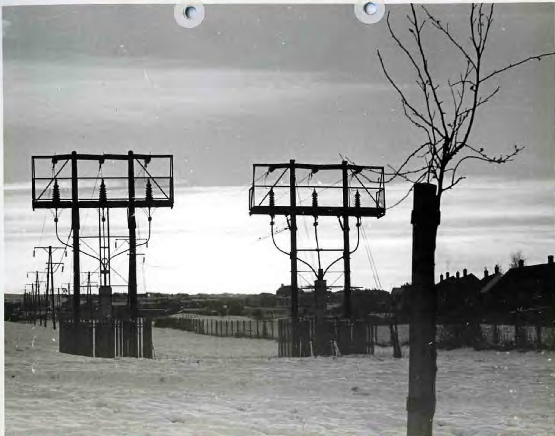
POWER LINES TO HEWORTH COLLIERY. FROM HIGH LANES. 1974
