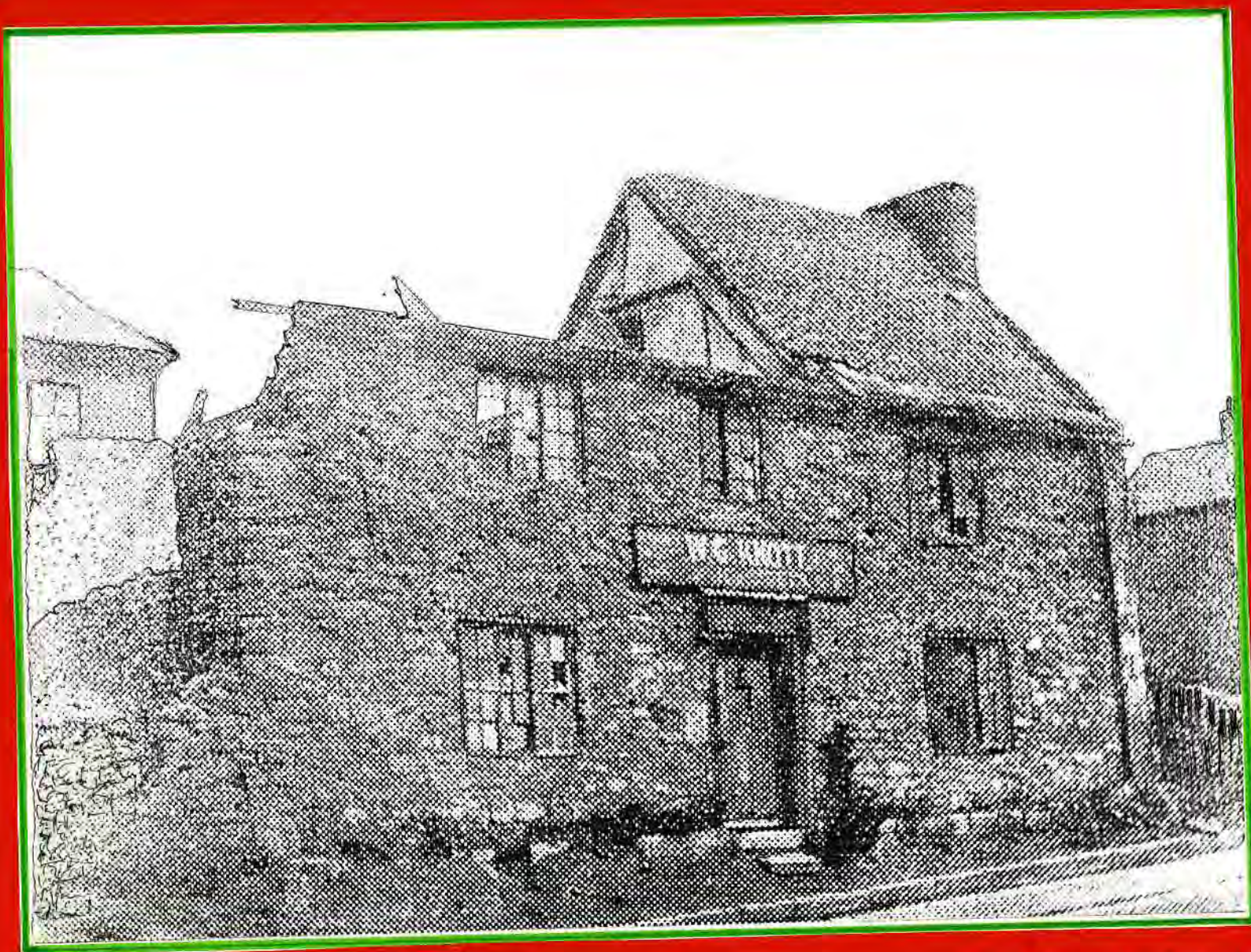
NETHERFARM. DERELICT AND IN USE AS A WORKSHOP AND STORE BY THE WILLIAM KNOTT, BUILDER. SAID TO BE THE OLDEST HOUSE LEFT IN HEWORTH VILLAGE AT THE TIME OF THIS PHOTO - C 1932. MR. KNOTT ONCE FOUND A FRENCH COIN DATED 1631 IN THE GARDEN. NETHER HOUSE WAS BUILT ON THE SITE IN 1937.
