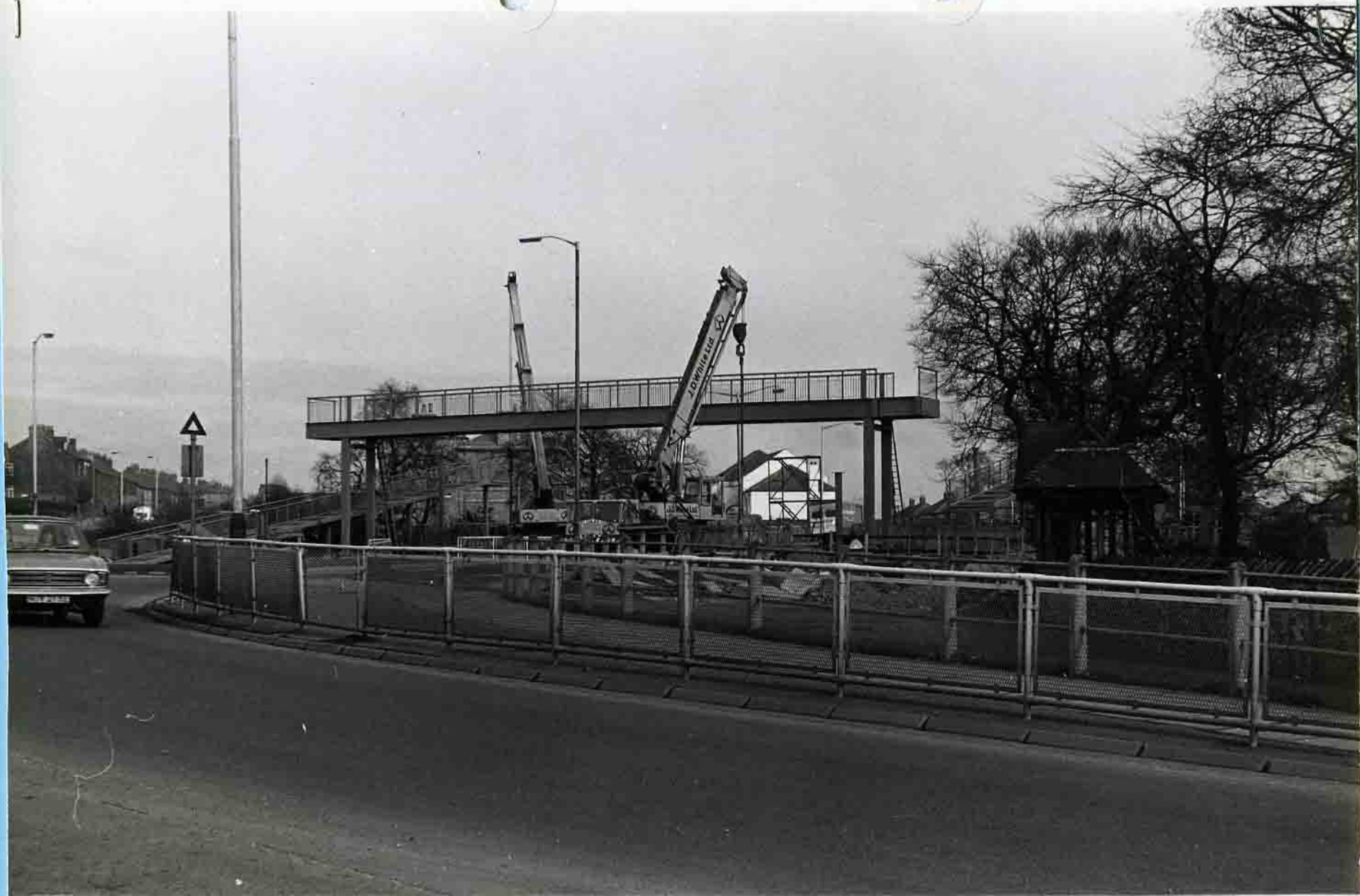
Building the footbridge at Heworth Roundabout 1973.
