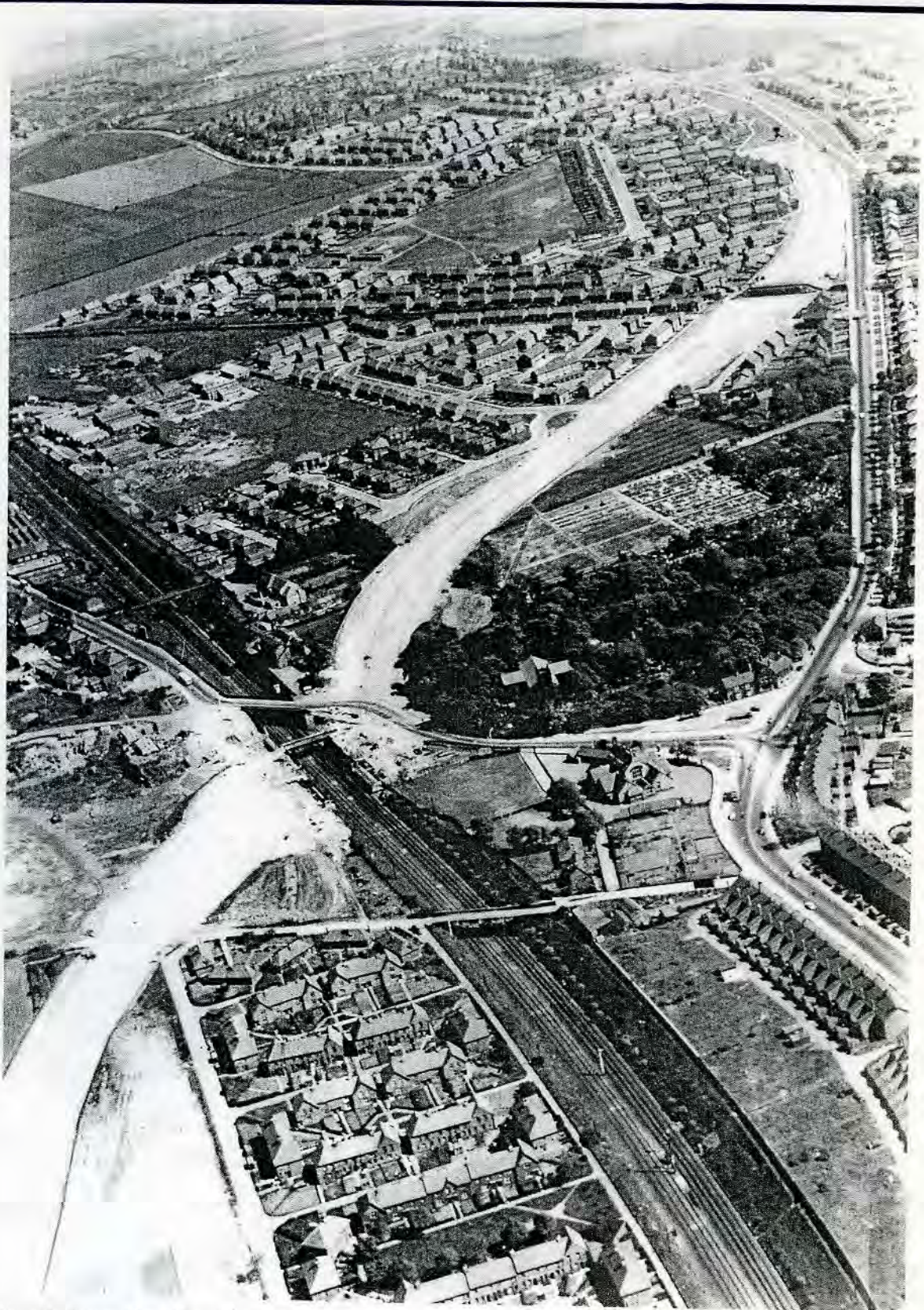
65. The first section of the £1½ million Gateshead-Felling bypass in May 1959. On the left of the photograph are Pelaw railway station and the C.W.S. factory at Pelaw.
