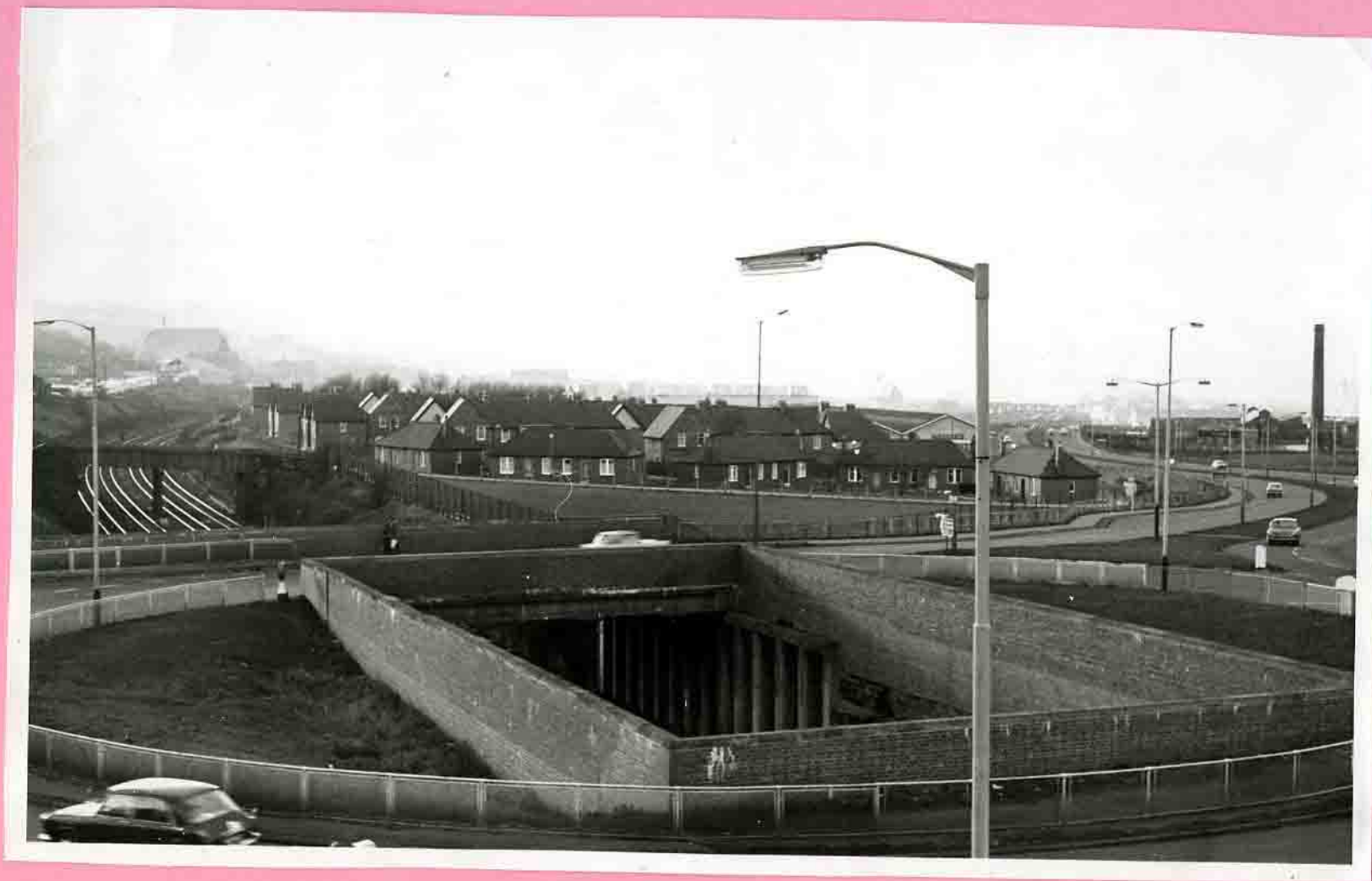
THE FIRST ROUNABOUT AT HEWORTH, CONSTRUCTED 1958-59 ON THE SITE ONCE OCCUPIED BY THE OLD HEWORTH PARSONAGE (1837), THE SUNDAY SCHOOL (1912), OLD COTTAGES ON THE EDGE OF HEWORTH DENE, AND THE BRIDGE OVER THE RAIL- WAY, CARRYING SHIELDS ROAD THROUGH HEWORTH VILLAGE TO PELAW. PHOTO: K. HEWITT.
