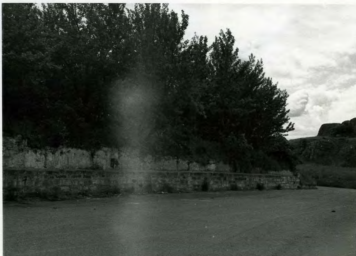
STONE BOUNDARY WALL (WESTERN END) OF NEST HOUSE AT FELLING SHORE. ROAD IN FOREGROUND IS NEW.
