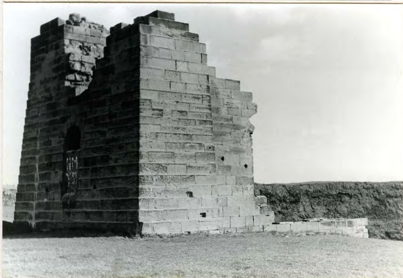
VIEWED FROM SOUTH. NOTE "TANK" ON RIGHT ie. CHEMICAL WASTE PHOTOS K. HEWITT
