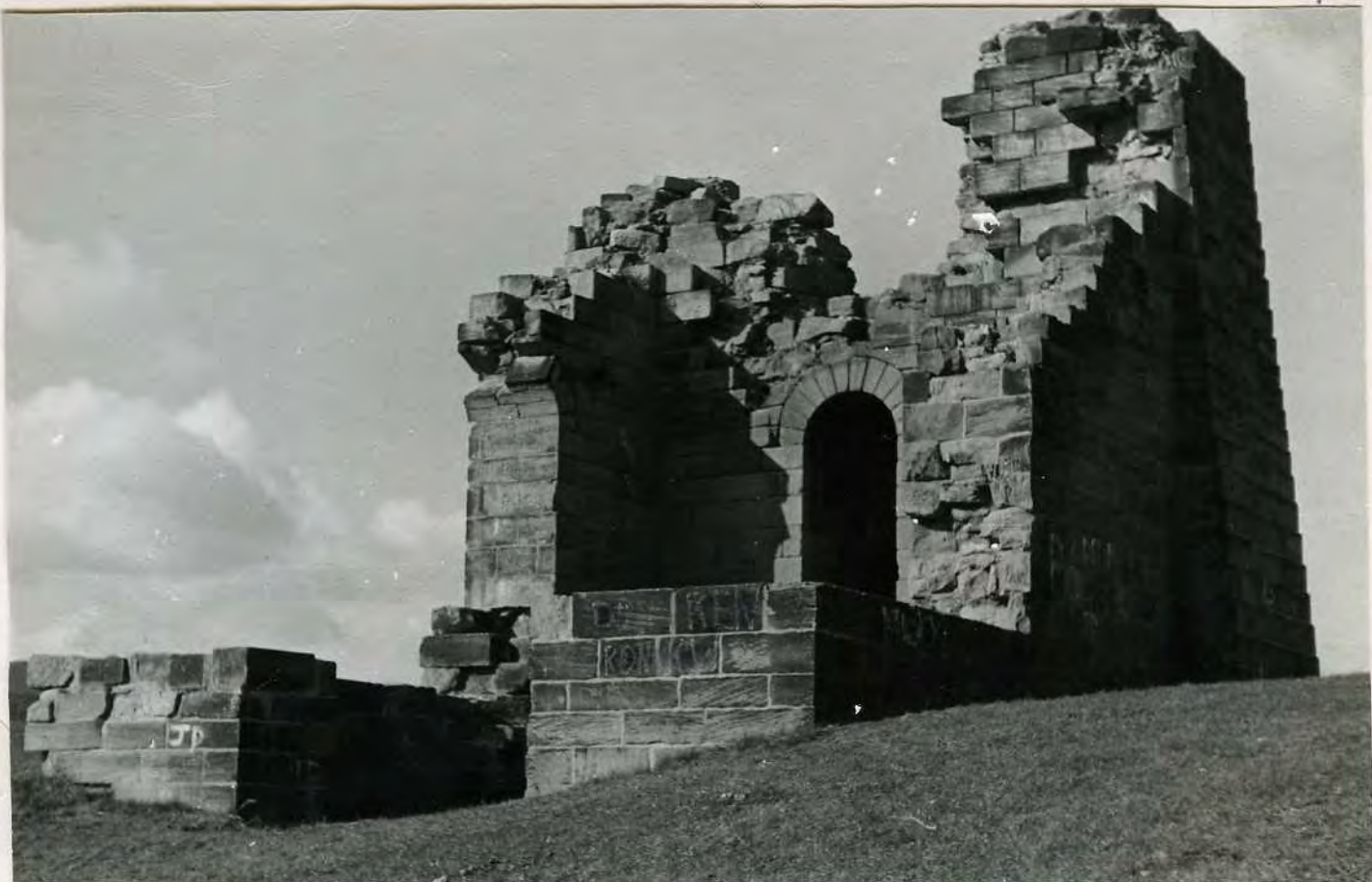
PRESERVED REMAINS OF FRIAR'S GOOSE COLLIERY ENGINE HOUSE. SEE THIS EASTON OF NEST HOUSE & FRIAR'S GOOSE PUMPING ENGINE.
