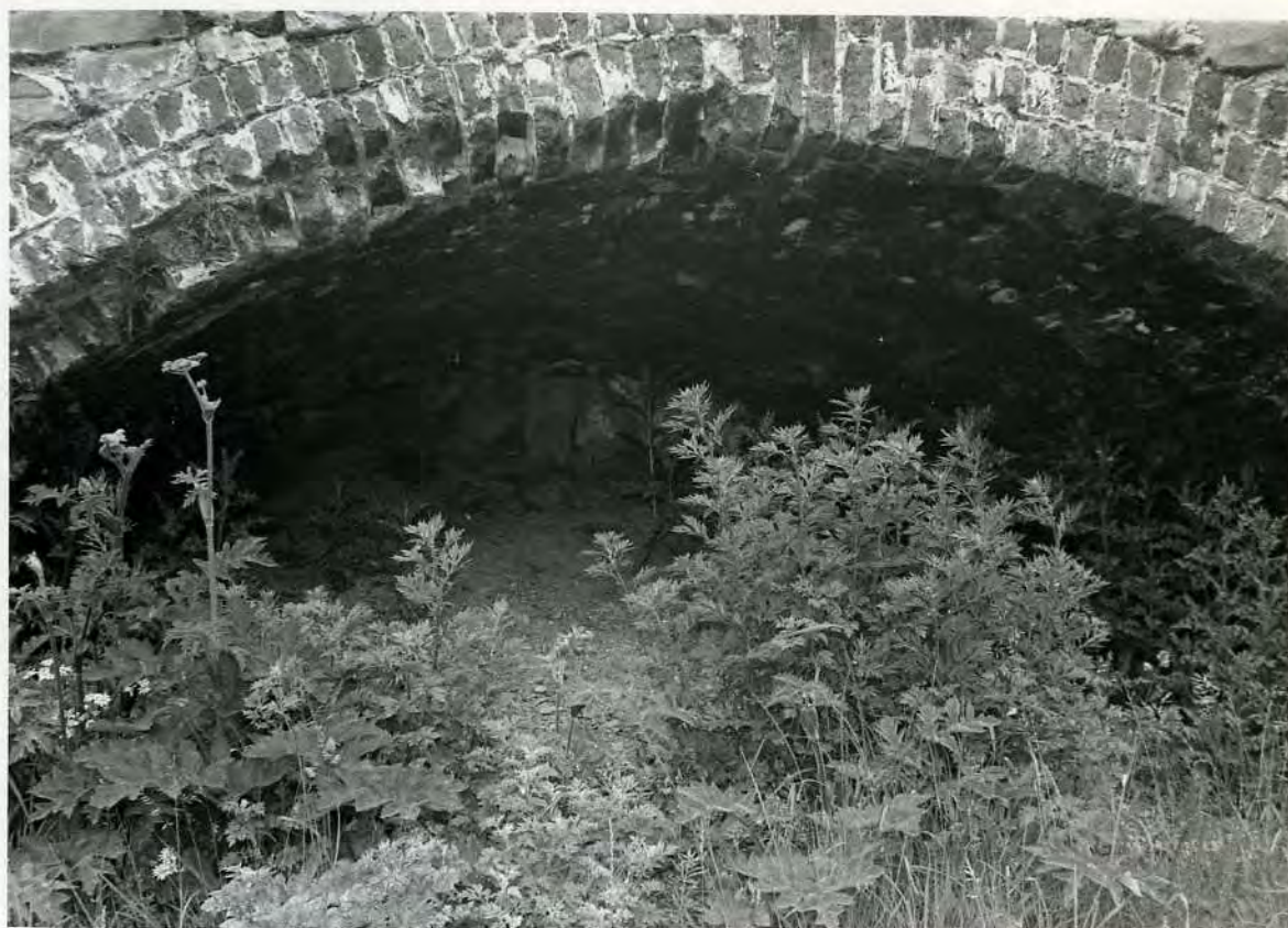
CHOSE UP OF TUNNEL EXIT ARCH ABOVE.
